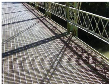
Steel grating bridge decks
